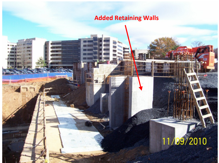
Figure 4: Added Retaining Walls to Allow for Backfill Prior to Pier Placement
